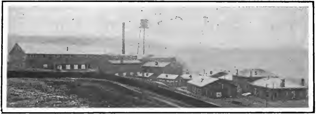
American Vanadium Co.'s plant near Bridgeville, Pa. 1—Ore storage building. 2—Furnace building. 3—Reduction building. 4—Crusher building. 5—Office and alloy building. 6—Storehouse. 7—Machine shop. 8—Carpenter shop. 9—Blacksmith shop. 10—Brick storage building
